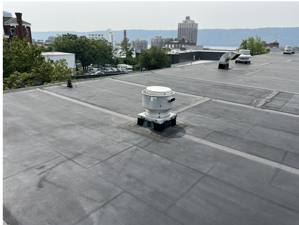
3 PHOTO 2 - ROOF LOOKING SOUTHWEST SCALE: N.T.S.
